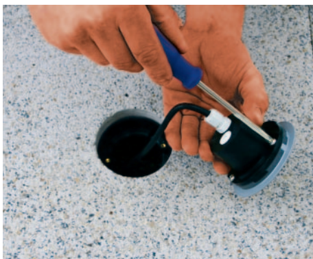
Step 4 Screw the diffuser and mounting ring to the inner casing.
